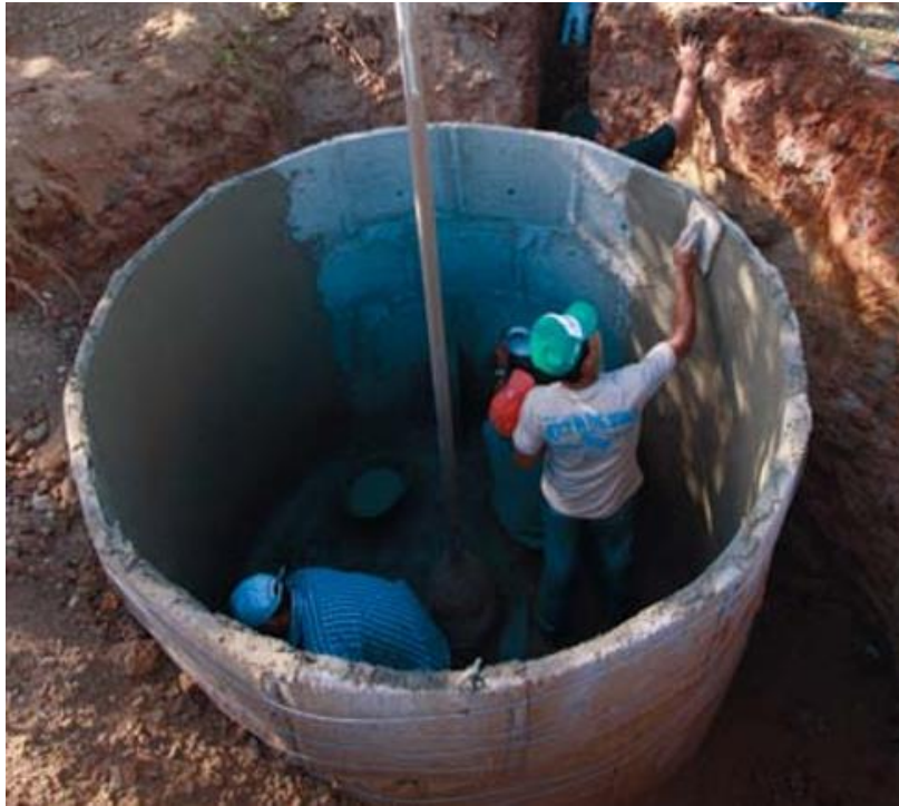
Figure 6. Construction of the digester walls with cement slabs, galvanized wire and plaster [5].
